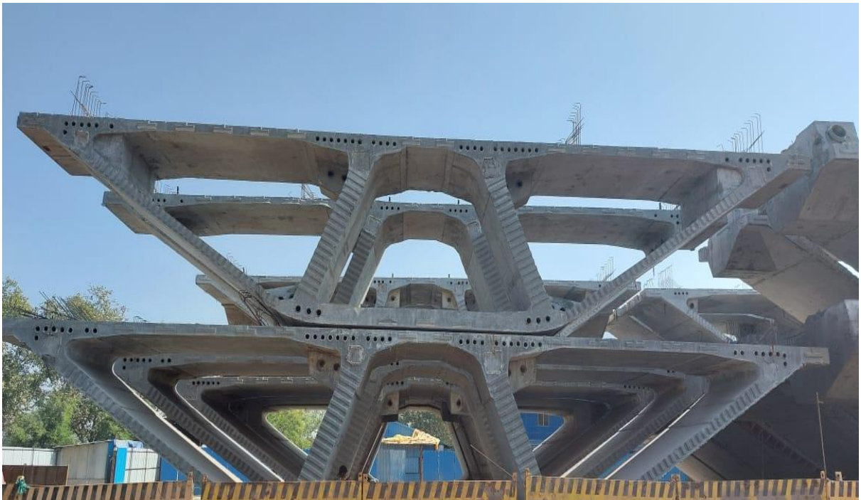
Stacking of Segments
