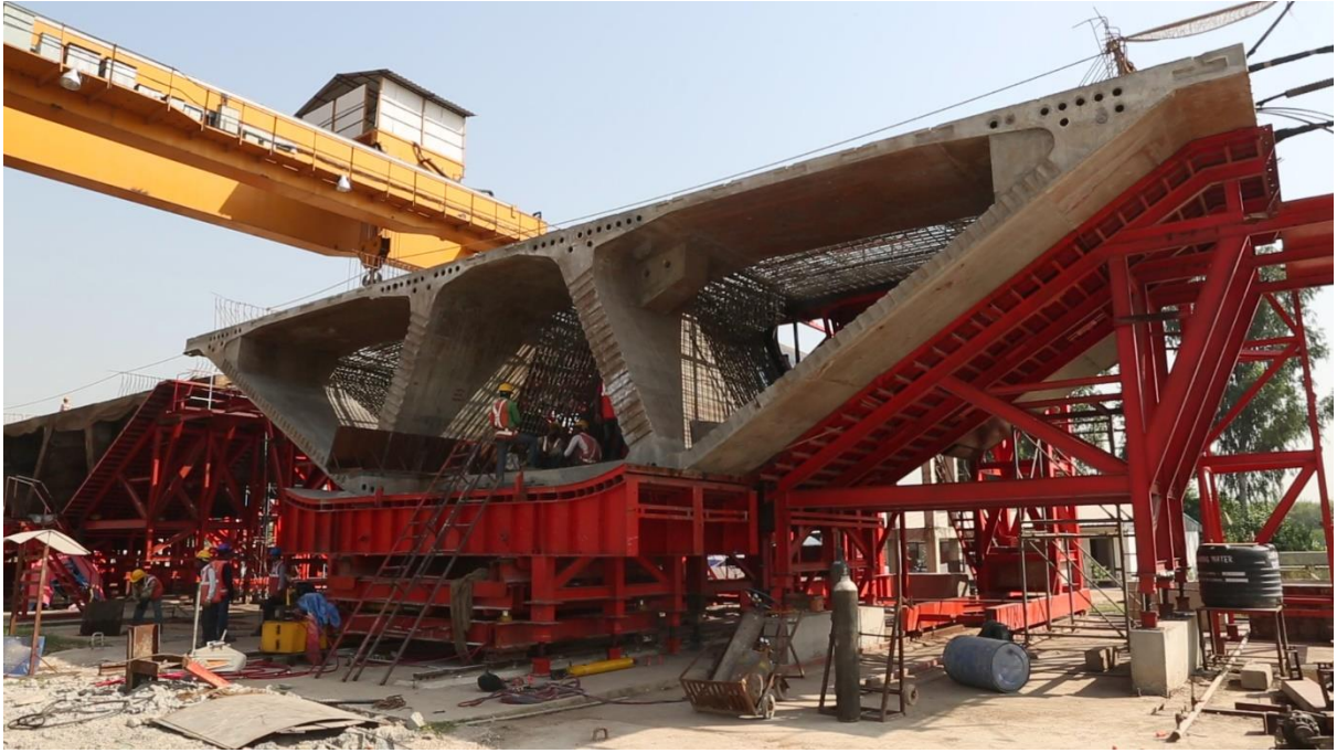
Casting of Segments
