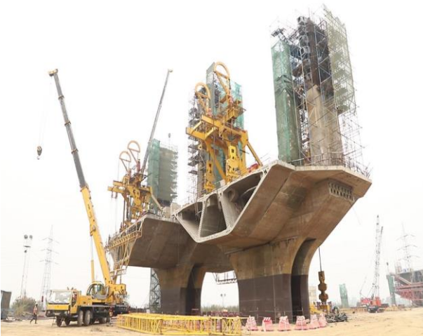
Construction of Piles
