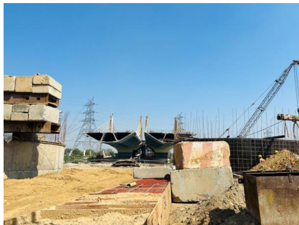
Construction of Coffer Dam
