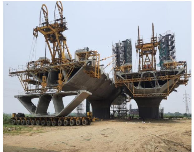
Installing Segments on piles
