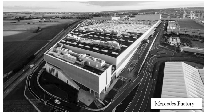
Figure 2. World’s first captive 5G mobile network has been installed for automobile production over an area of more than 2 million square feet.
