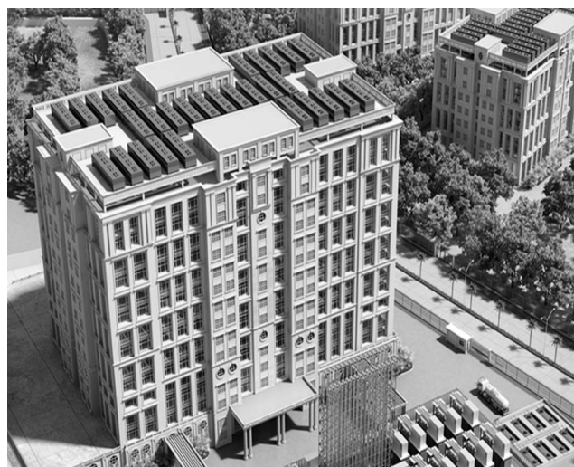
Figure 1. India's largest Data Center building, Yotta NM1, Navi Mumbai.
