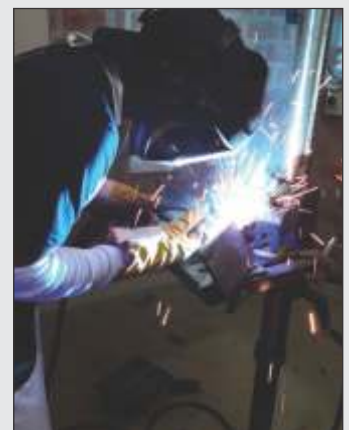
Contestant performing welding in 2F position
