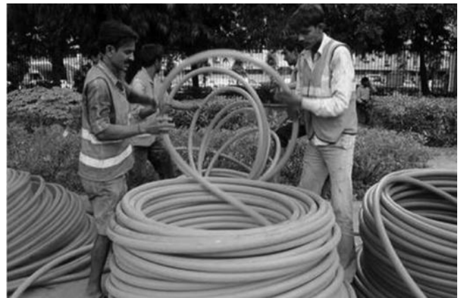
Figure 1. Bharatnet is the world's largest rural connectivity program using optical fibres to provide broadband facilities to 2.5 lakh gram panchayats.
